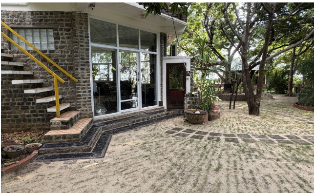
Path and entrance landscaping in progress
