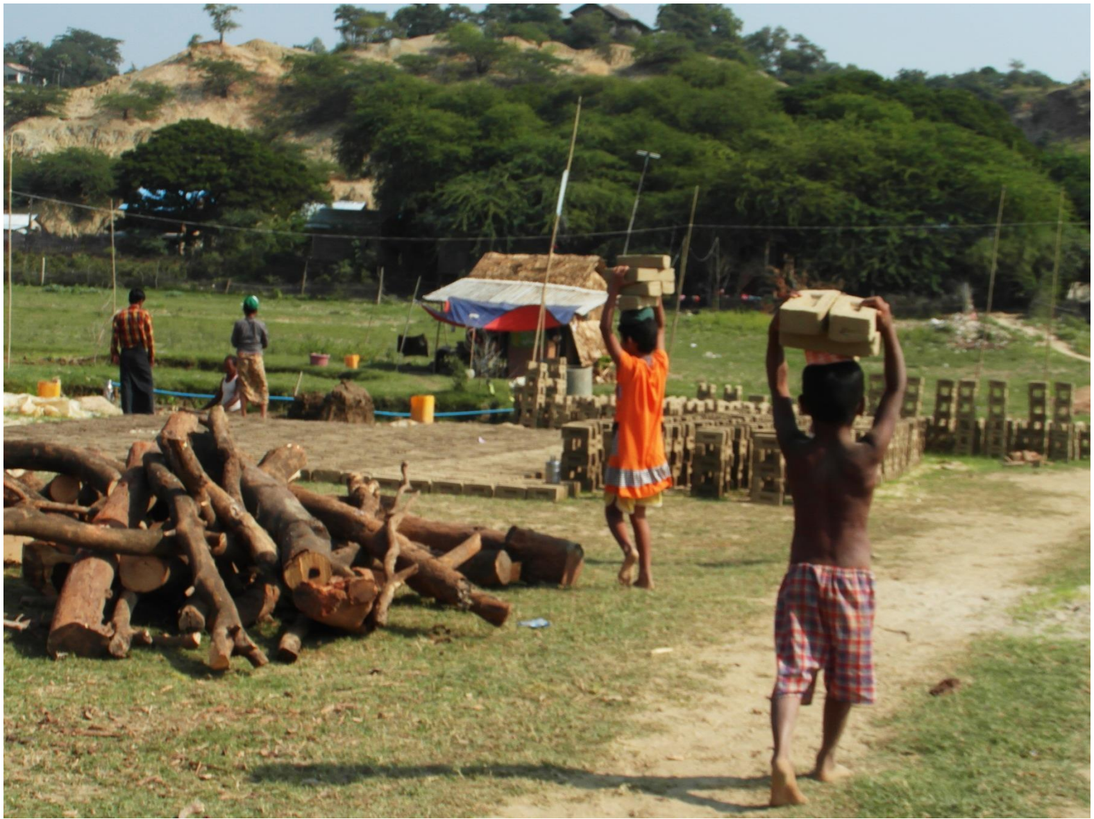
Young helpers carry the bricks ...
